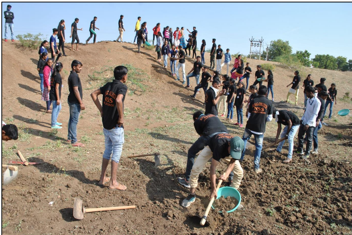
The NSS team Preparing Village Road 8 Dec 2020
